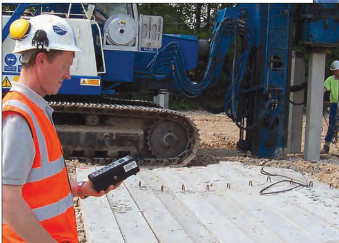
E-Saximeter with antenna receives energy and depth data from wireless transmitters.
