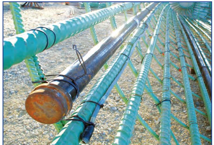
Thermal Wire™ attached to rebar cage (shown adjacent to access tubes.)
